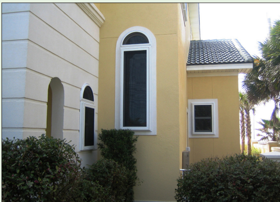
Figure 4-8: In-place stainless steel impact screen protects several windows of a coastal residence. This system requires no deployment and provides shade. (Source: Roll-a-way/QMI)
