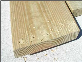
Using galvanized or treated deck screws, screw the boards together using the cordless drill with the appropriate screw driver bit.
