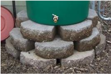
Figure 2: A rain barrel is placed upon stacked blocks to help increase flow rate from the barrel and increase accessibility to the spigot.
