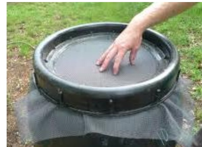
Figure 3: A fine wire mesh atop the rain barrel helps prevent mosquitoes from inhabiting the stored water.
