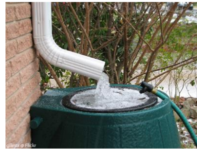
Figure 1: A downspout is modified to drain into a rain barrel rather than to the landscape. A simple modification that can easily be completed without much experience or skill. .
