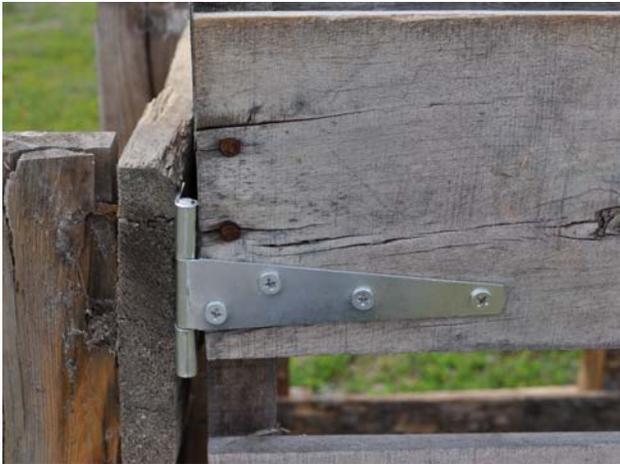
6. Attach the hinges to the top and bottom of the inside of the compost bin. Try to put as many screws as possible into the pallet's frame. Set the front pallet on the bricks and attach the hinge to the front pallet (shown left).
