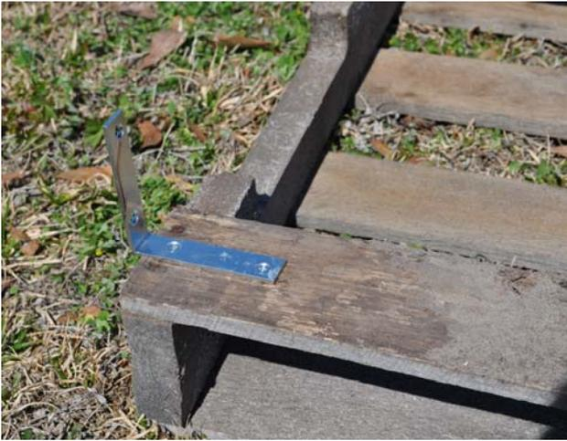
3. Attach both the top and bottom L brackets to the inside of the side pallet first (shown left). Then stand the pallets back up and attach the L brackets to the back side of the back pallet (shown below).
