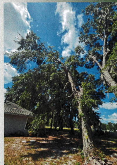
Compromised tree structure overhanging the house.
