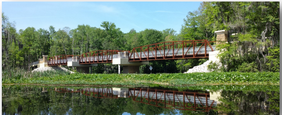
Dunnellon Trail Bridge
