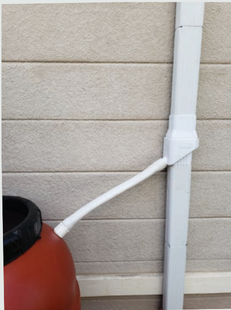
These downspout diverters are installed in line with the downspout. A portion of the rainwater flow will be diverted to the rain barrel through the hose attachment. Some come with built in screens to keep out debris.
