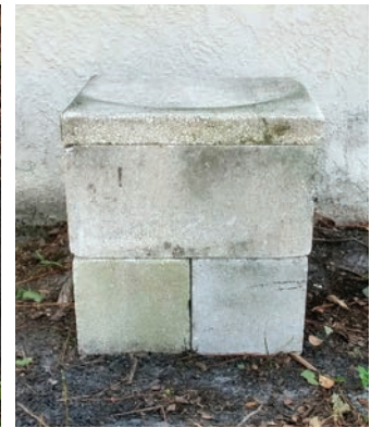
A flat paver stone can be placed on top of stacked block for added stability.
