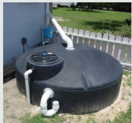
Examples of larger rainwater collection systems: left, 500 gallons each; center, 2,000 gallons; above, 1,000 gallons (partially buried)
