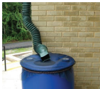
For sealed-top barrels, cut a hole for just the downspout or remove the entire top, then cover with screen to keep out debris.
