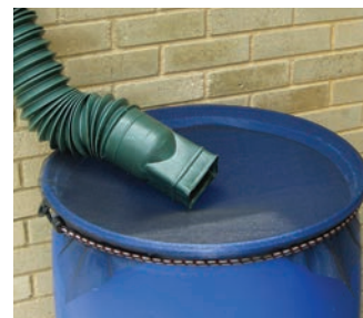
For sealed-top barrels, cut a hole for just the downspout or remove the entire top, then cover with screen to keep out debris.
