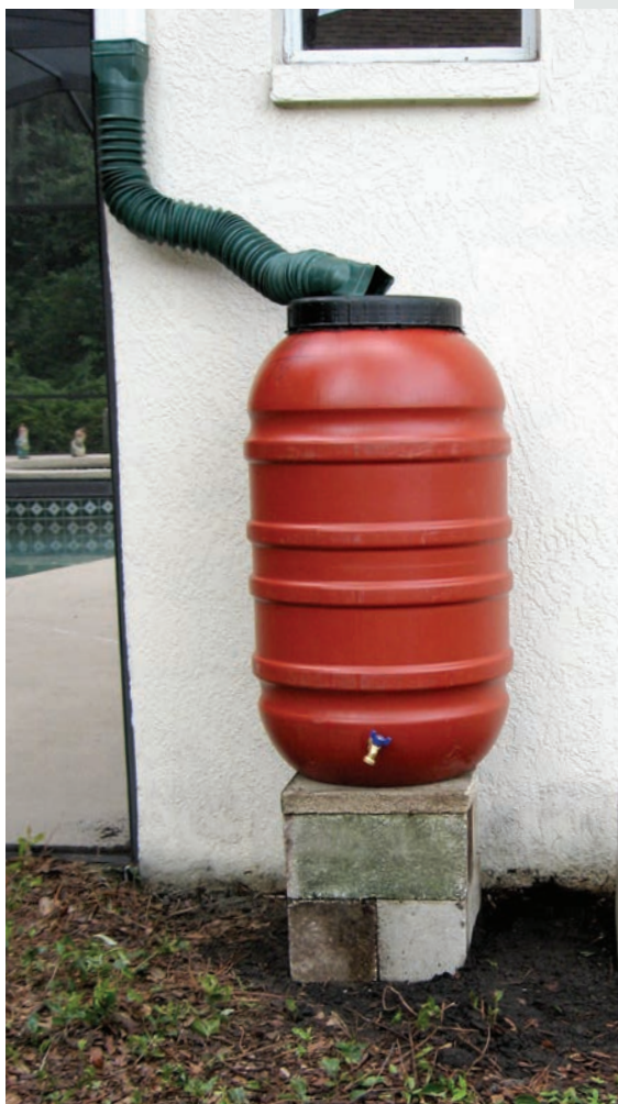
Place the barrel on top of blocks and place the gutter attachment on top of barrel opening.
