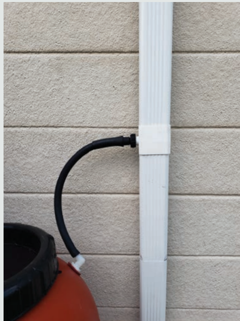
These downspout diverters are installed in line with the downspout. A portion of the rainwater flow will be diverted to the rain barrel through the hose attachment. Some come with built in screens to keep out debris.
