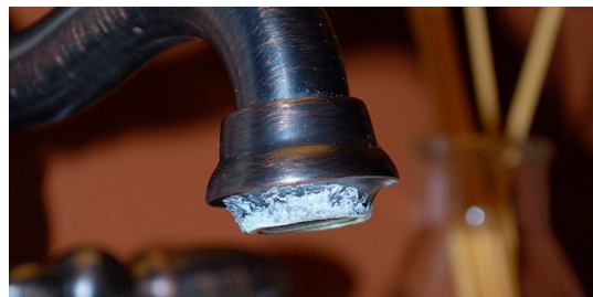
Calcium Buildup on a Faucet. Source: Mr. Rooter
