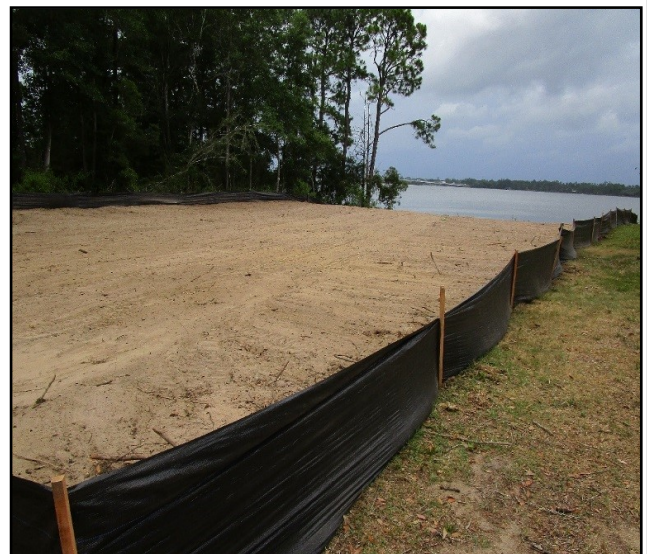
Figure 1. Vacant lot being prepared for building upon. Photo: M. Burba
