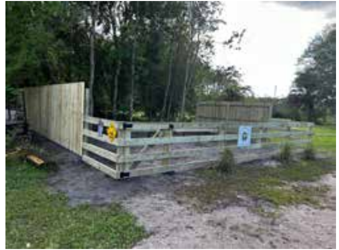
SJC Beekeeper's Apiary renovation project
